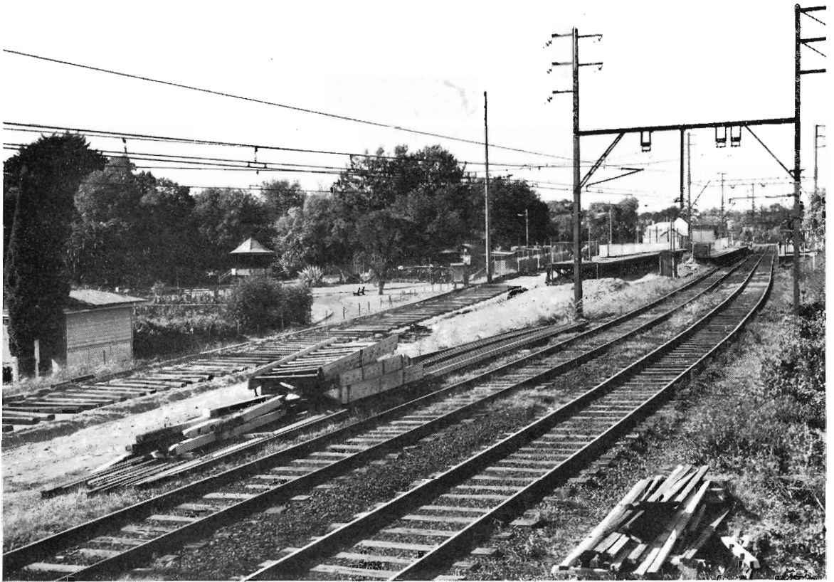
Canterbury station showing (at left) sleepers in position for temporary track.
