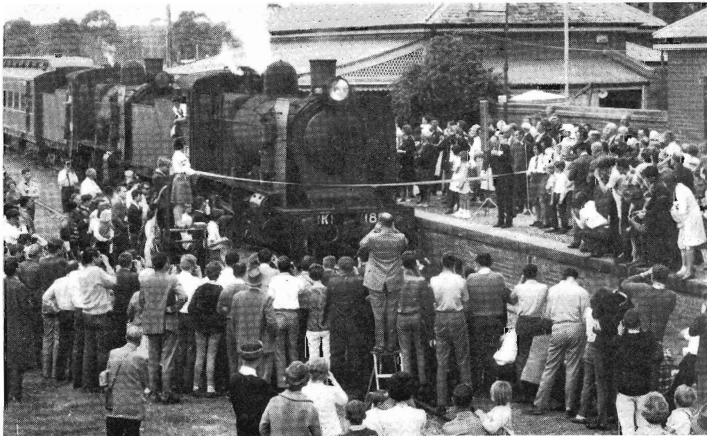
RE-OPENING: At Avoca, on October 29, the Shire President, Cr. M. W. Dawson, cuts the ribbon for the re-opening of the line to Ararat. Organized by railway enthusiasts, it was the occasion of the first revenue train to use the line since July 1959, when the line was closed for economic reasons. (A. R. E. photograph)
