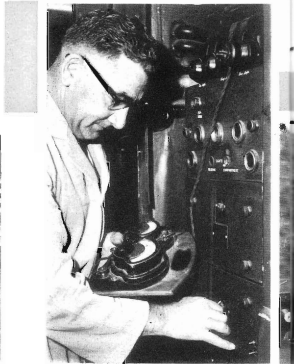
Electrical Mechanic J. Neve checks electrical load on carriage.
