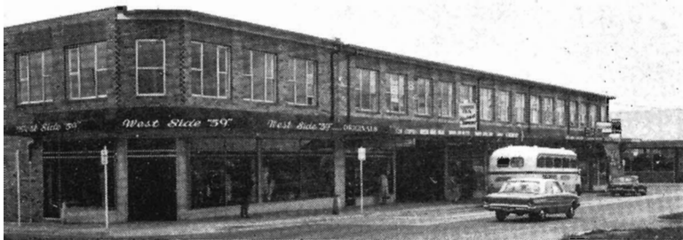
Part of shopping development at Glen Waverley
